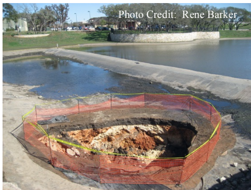
Figure 7. Collapse of a water treatment lagoon in Texas, which was caused by the weight of the overlying water breaching the approximately 1 foot protective seal. Catastrophic collapses in karst are not uncommon.
